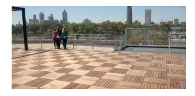
Maximo Deck Tiles are also an excellent option for conventionally constructed decks. Simply double your stringers 24" on center and fasten them down at the corners with 4 Pro Plugs per tile. Maximo deck tiles provide a unique appearance while also significantly lowering overall construction costs. Deck tiles can be installed to create various designs and patterns.
